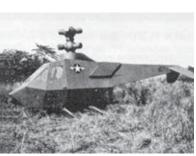
This was an attempt by Sikorsky to build an armored helicopter as opposed to adding armor to sensitive areas of the fuselage. The concept projected some 1,800 pounds of armor on a 6,800 pound aircraft. Subjected to heavy ground fire in late 1970, this aerial armadillo was merely dented by armor-piercing and ball ammunition. Bell's UH-1 Iroquois joins the L-4 Cub
