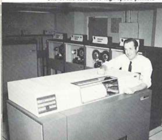
One of two IBM 1403 high speed printers ↓
