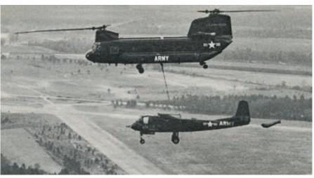
An Army CH-47 Chinook is shown airlifting an AO-1 Mohawk during operations of the 11th Air Assault Division conducted at Fort Benning, GA. Carried by sling load, the Mohawk is flown straight by means of the 'sock' at its tail.
