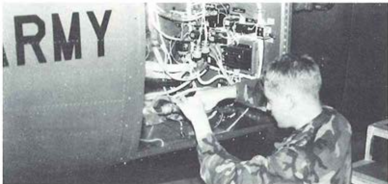
TROUBLESHOOTING AN AH-1S ELECTRICAL SYSTEM
