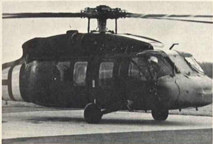
The UH-60A Black Hawk is shown after an artificial icing flight
