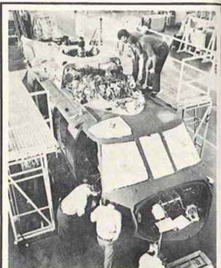
A UH-60A Black Hawk helicopter is shown in its final assembly phase on the Sikorsky Aircraft production line at Stratford, CT.
