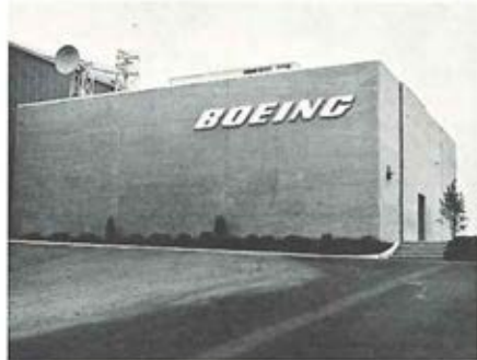
BV Flight Test Facility
