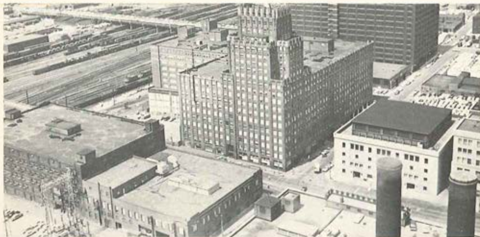
MART BUILDING, ST. LOUIS, MO.
