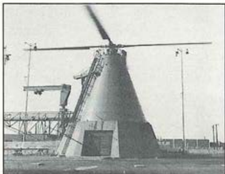
Fiberglass rotor on whirl tower
