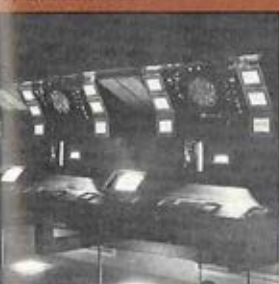
Direct communication with 29 sites at Ft. Rucker, and 20 frequencies for communication with aircraft are provided by each of the four radar scopes at Hub Control in Cairns Army Airfield. Serving aircraft within a radius of 50 miles of Ft. Rucker, Hub Control is expected to service over 100,000 requests for advisory service during 1971.
