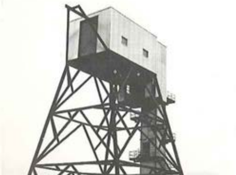
9. We have the only heavy-lift hoist test facility that can test a 30-ton load at 2\frac{1}{2} g.
