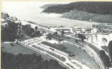
An aerial view of AVLABS
