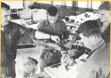
A technical representative is shown instructing the maintenance personnel of the 1st Cavalry Division's 1st Squadron, 9th Cavalry, in the workings of the new OH-6A Cayuse observation helicopter. The aircraft has just arrived in the Cav Division for service with the reconnaissance unit.
