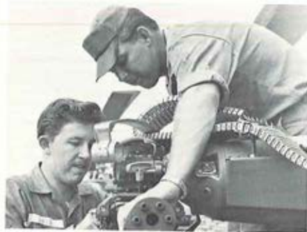
SPECIALISTS Tony M. Ross (left) and Jack A. Smith, with the 1st Aviation Brigade's 334th Armed Helicopter Company, prepare one of their new rapid-firing miniguns. Just being received in Vietnam, the weapons system closely resembles the Old Gatling gun in that it employs six rotating barrels.
