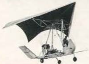
FLEX WING STOL "FLEP," popular name of the easy-to-fly XV-8A, is under study by Army's Transportation Research Command as an aerial "truck," capable of operating out of rugged areas.
