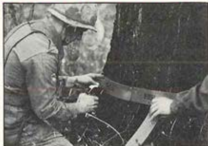
Men from the 127th Engineer Battalion, 11th Air Assault Division, rappell down 120-foot nylon ropes into a heavily wooded area (top left); affix demolition charges to the larger trees (top right); use chain saws and other demolitions to clear the area in minutes (bottom left); and watch as an Iroquois helicopter lands on the 'Instant Helipad' within minutes after site selection. (USA photo).
