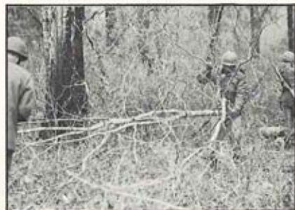
Men from the 127th Engineer Battalion, 11th Air Assault Division, rappell down 120-foot nylon ropes into a heavily wooded area (top left); affix demolition charges to the larger trees (top right); use chain saws and other demolitions to clear the area in minutes (bottom left); and watch as an Iroquois helicopter lands on the 'Instant Helipad' within minutes after site selection. (USA photo).
