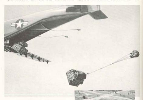
The Caribou's slow speed under full control, and straight-out rear exit permits accurate delivery and close grouping of logistic supplies.
