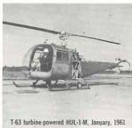
T-63 turbine-powered HUL-1M, January, 1961
