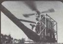
Microwave station on 4,000' ridge; all 8 tons material; 2 days flying.
