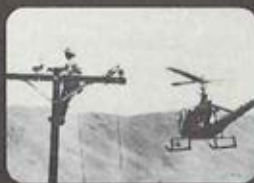
2½ mile powerline built in 6 hrs., 50 mins. with E's 305 hp at work.
