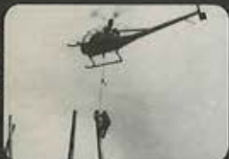
12E, first light copter to erect entire powerline; 40' poles, el. 5,000 ft.
