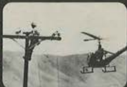
2 1/2 mile powerline built in 6 hrs., 10 mins. with E's 305 hp at work.
