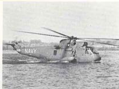
Flown for the first time in late March at Sikorsky Aircraft Division's Stratford, Conn. plant the Sikorsky HSS-2 features a boat hull and twin gas turbine engines. Having all-weather capabilities, the world's largest amphibious helicopter will be added to the Navy's anti-submarine weapons system. Sikorsky has been awarded a $32 million Navy contract for the development and manufacture of the HSS-2.
