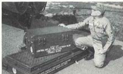
Ready to unpack the portable X-ray equipment used in inspecting aircraft at Fort Benning, SFC Patrick E. Pettingill assists in the new method of inspecting aircraft component parts while they remain intact. (U.S. Army photo).
