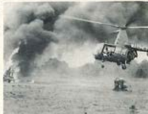
3. Flying to the crash scene, the HOK hovers and sets the fire apparatus on the ground automatically.
