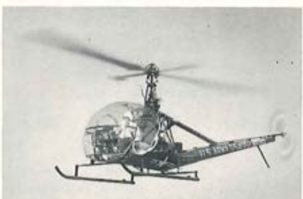
The H-23D, incorporating new sturdy transmission and drive system.
